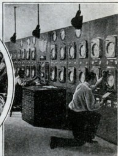
The central tower, or RCA building, is 70 stories high, rising 836 feet above the street. The view shown is taken from the garden on the roof of one of the skyscrapers adjoining the group. Center shows a maze of wires, the hooking of which was a major feat in itself. Right shows air control boards which supply changed air to the studio floors, which have no windows.
